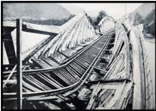
Destroyed railway bridge in Otta, Norway. Taken after German occupation in 1940
